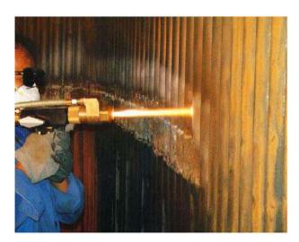
High chromium content nickel based alloy Cr3C2-NiCr & In presence of sulfur and vanadium atmosphere NiCrTi & amorphous alloy of FeCrBSi as a widely used corrosion & wear resistant coating material, possesses good ability against oxidation, sulfur induced corrosion and hot corrosion.
